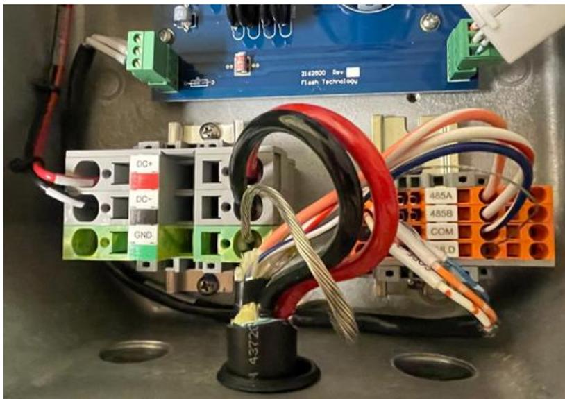
Figure 2-8 – Flashhead Cable Terminal Block
