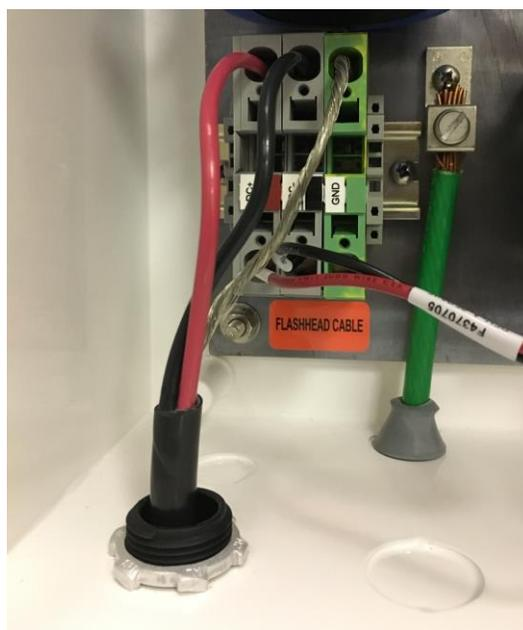
Figure 2-5 – SC 370 Flashhead Cable Connection
