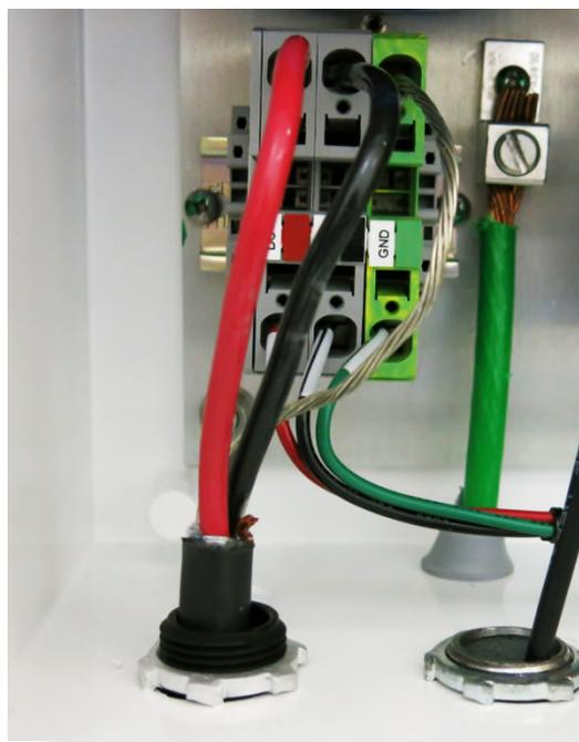
Figure 2-5 – SC 370 Flashhead Cable Connection
