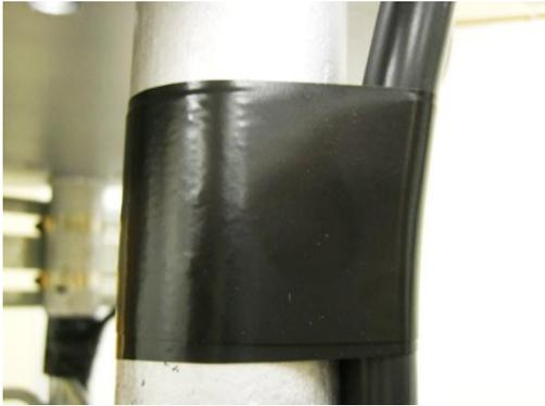
2. Wrap three full turns of one-inch Scotchrap Filament #890 tape, or the equivalent, over the Scotchrap #50 tape.
