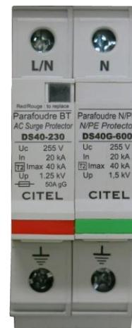
Figure 1-1 – AC Power Surge Suppressor Assembly
