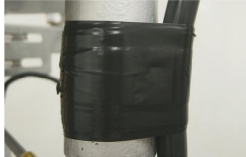
4. Perform steps 1 through 4 also directly above and below any tower leg flanges that the cable may cross. The cable should be spaced approximately 1 inch from the edge of each flange.
