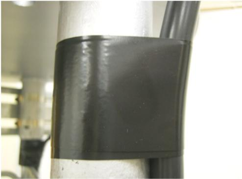
2. Wrap three full turns of one-inch Scotchwrap Filament #890 tape, or the equivalent, over the Scotchwrap #50 tape.
